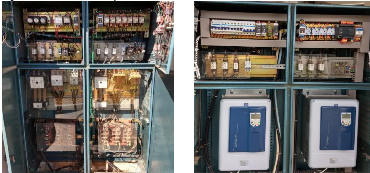
Figura 10: Painel sem CLP x painel com CLP
