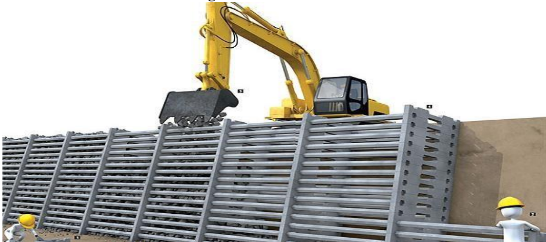
Figura 6 - CRIB-WALLS
